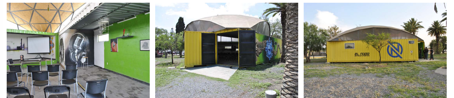
El Nodo, constructed and in operation since 2010
